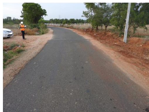
Narrow-curved road, Coimbatore Rural District
