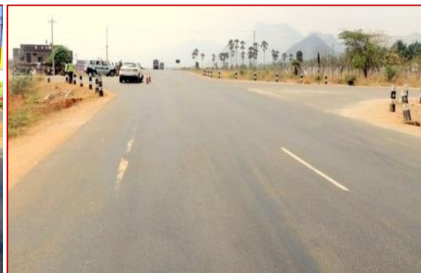
Typical intersection with no controls/signage (NH47 By-Pass, Vellalur junction)
