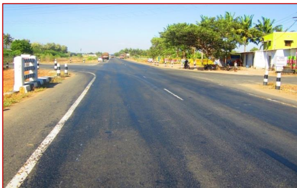
Typical intersection with no controls/signage (NH47 By-Pass, Pattanam Pudhur junction)
